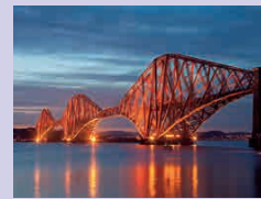
Forth Rail Bridge
